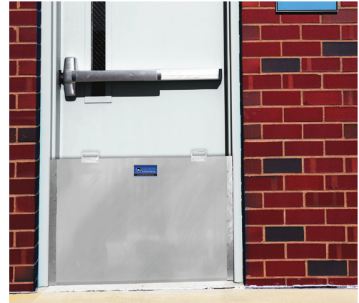
#5027MA mounted to the inside of the door frame.
