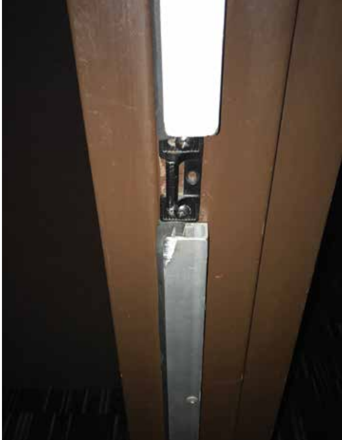
Figures 4 and 5 detail the results of poor specification and installation of hardware on an opening. The picture shows that the seal was notched out to accept the surface-mounted closer and the strike.
