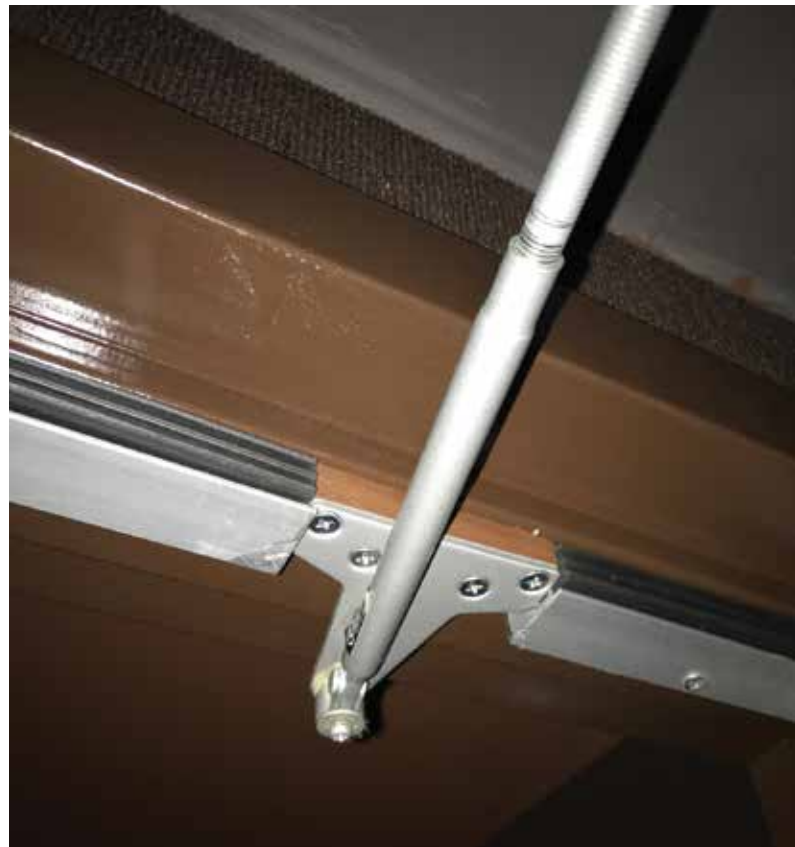
Figures 4 and 5 detail the results of poor specification and installation of hardware on an opening. The picture shows that the seal was notched out to accept the surface-mounted closer and the strike.
