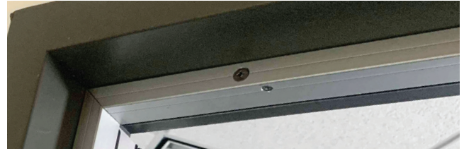
#5077CA Installed on head of frame.
