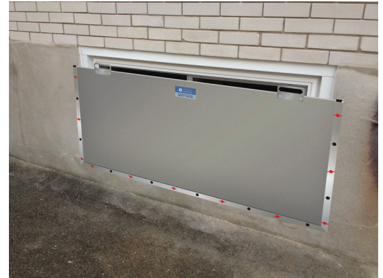
#5128MA mounted to a basement window.
